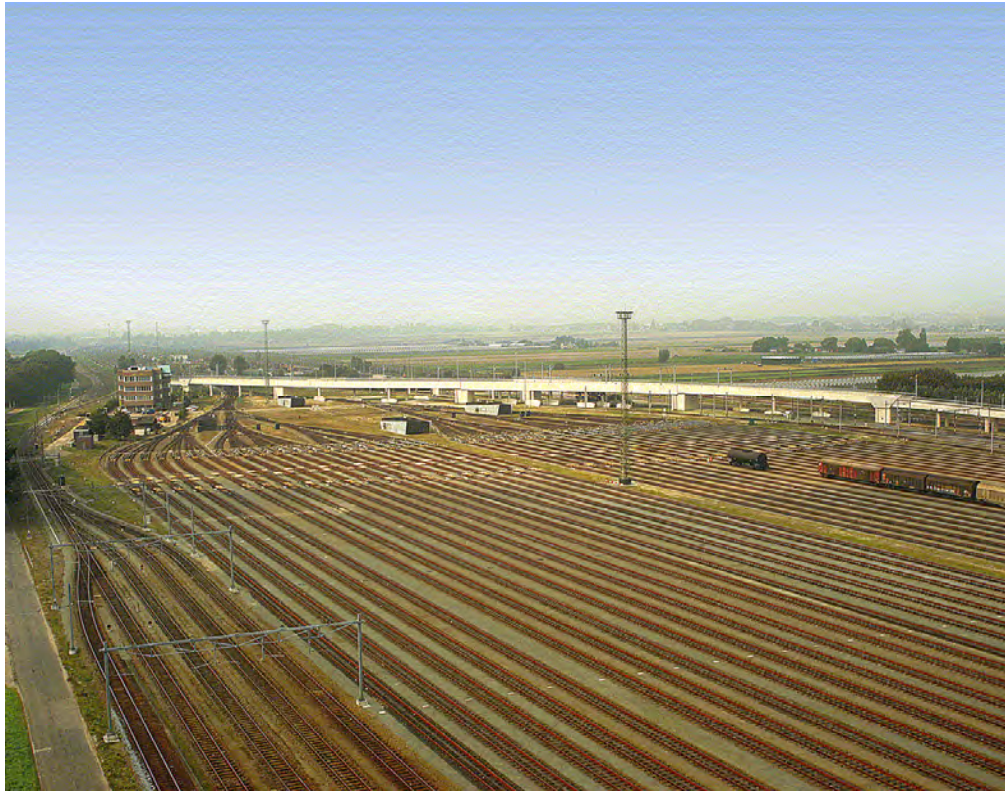
Figure 8. Crossing the railroads at 20 meter depths over 700 meters.
